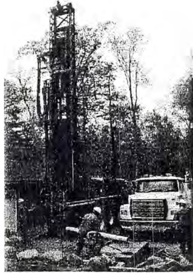
Vertical loop drilling in driveway
