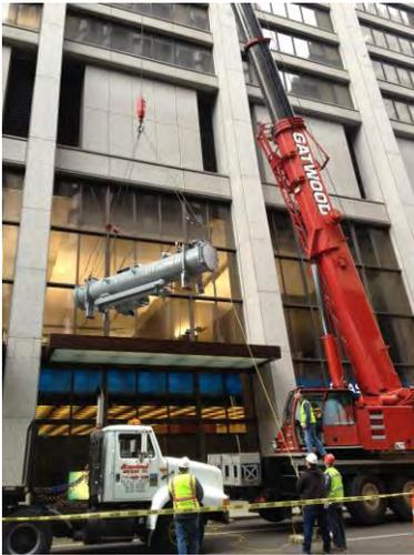
**Figure 9 Chiller being Hoisted through Building Louvers**
