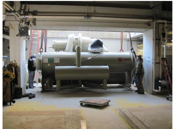
There is an oversized main header system with near net zero pressure drop in the middle of the campus that facilitates the control and sequencing of chillers. This new plant was designed at a highly efficient Integrated Part Load Value (IPLV) of 0.370. In addition, the new controls system eliminated the manual control of the chilled water plant and automatically operates the chillers, cooling tower, and pumps which were commissioned and functionally tested to ensure optimum energy efficiency.
