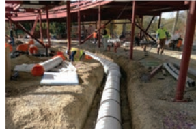
Image 2: Underground Ductwork
