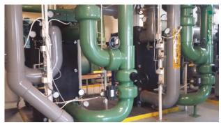
**Heating:** Three (3) natural gas-fired boilers each rated at 12.25 MMBtu generate hot water for comfort heating purposes. Hot water is generated between 180-185 °F and is used for comfort heating purposes. There are three (3) variable-flow hot water pumps each rated at 50-hp. The AHUs feature hot water coils; the FPBs feature hot water reheat systems that temper the primary air from the AHUs before supplying it to the conditioned spaces.
