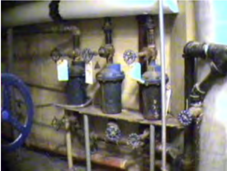
Leaking steam trap on the left
