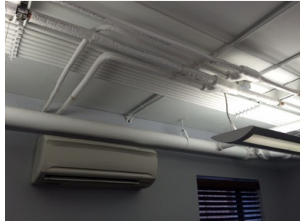
VRF Wall Mounted Evaporator
